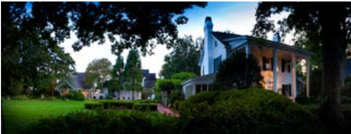
The front façade of the Fearington House Restaurant, with Inn rooms visible in background, left.
